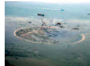
Construction of the Eastern Scheldt pilot scheme
