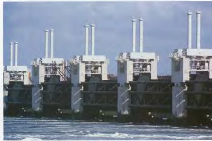
Fig. 8. The storm-surge barrier in open position. The steel gates in between the piers can be raised and lowered, but for most of the time they will be suspended above the waves. Photograph NIOO-CEMO, Yserck.
